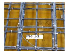
Application example: Embedded in reinforced concrete structure
